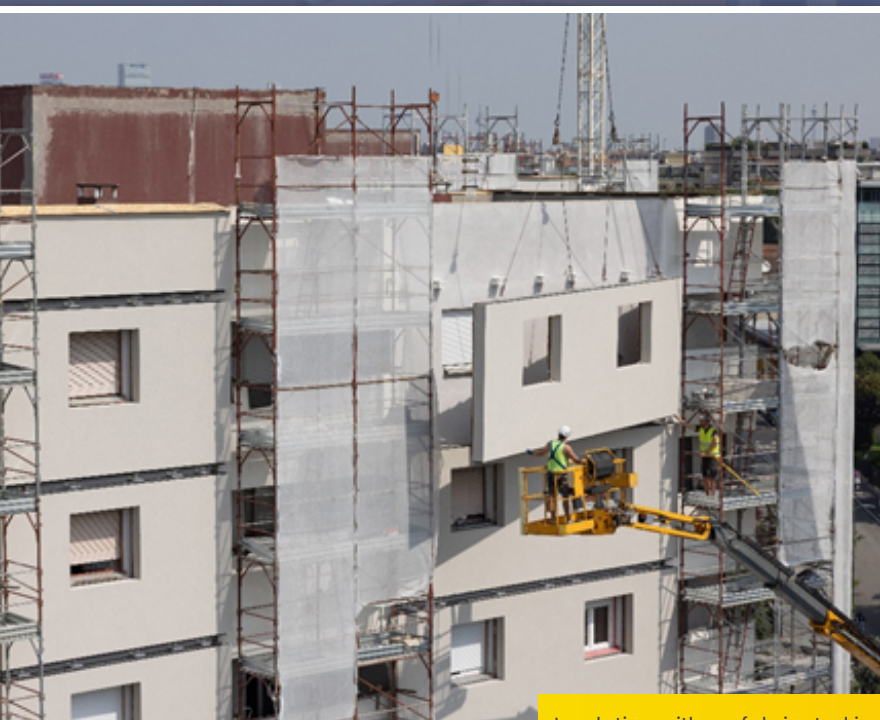
Insulation with prefabricated insulation panels made from rice by-products (© Ricehouse)
