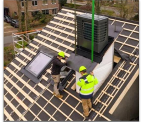
Modulised energy supply
